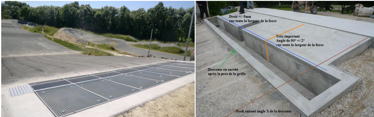
Figure 1: Photographs showing a safety start gate. This is the safest form of starting gate, and is retained on the site, totally flush.
